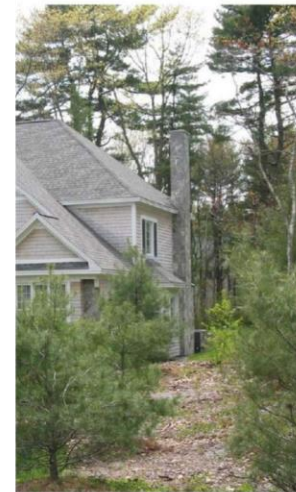
fig A. 23: Stone Chimney & HVAC Screen
